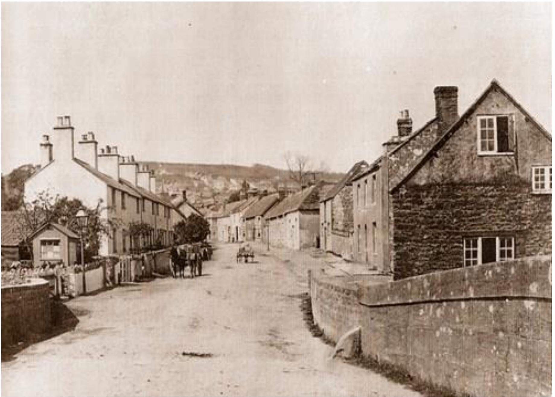
View from Bridge in 1890 showing Drill Hall before Gable added
