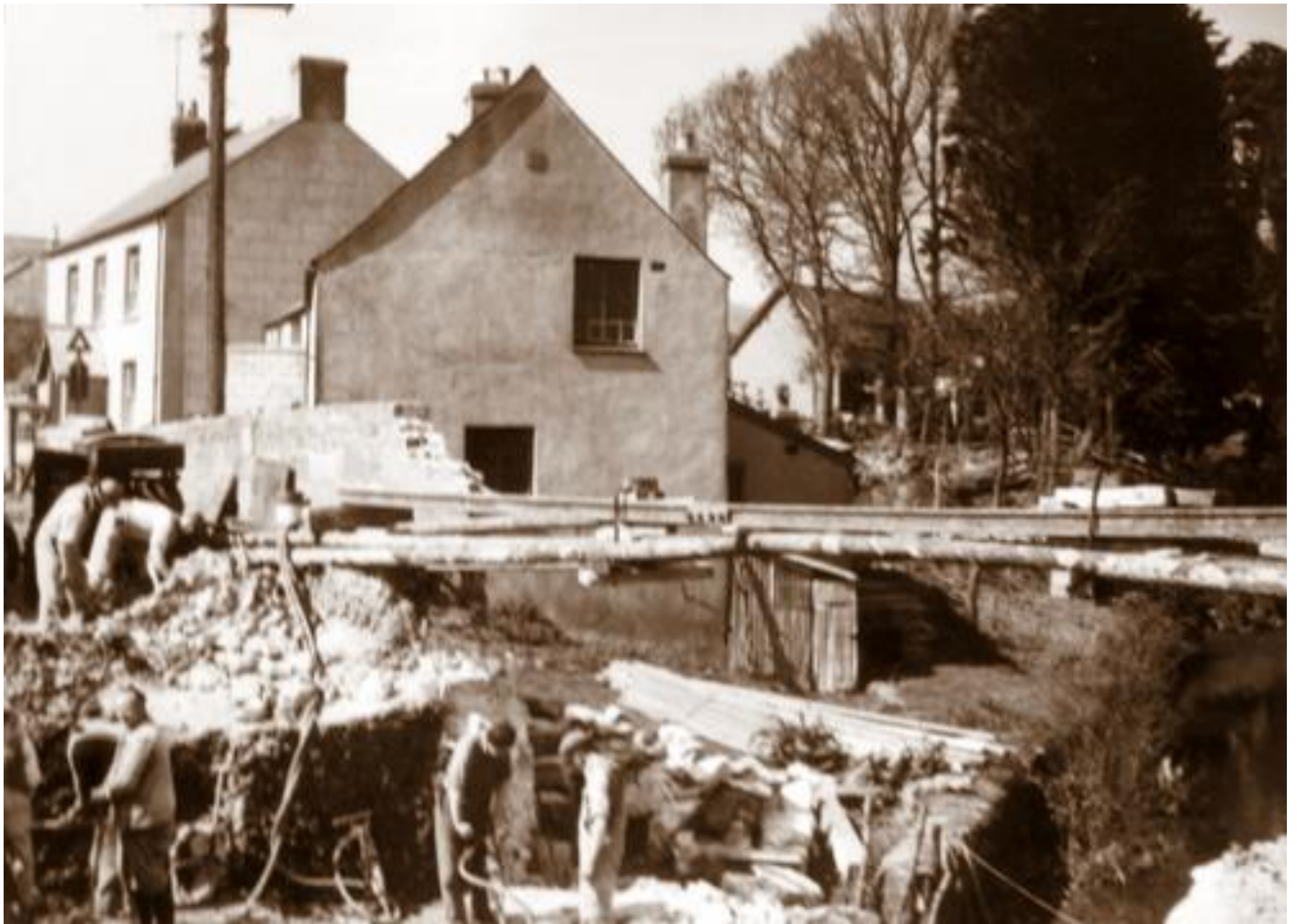
New Bridge in course of construction
