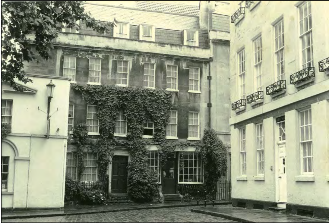
Elton House before work started
