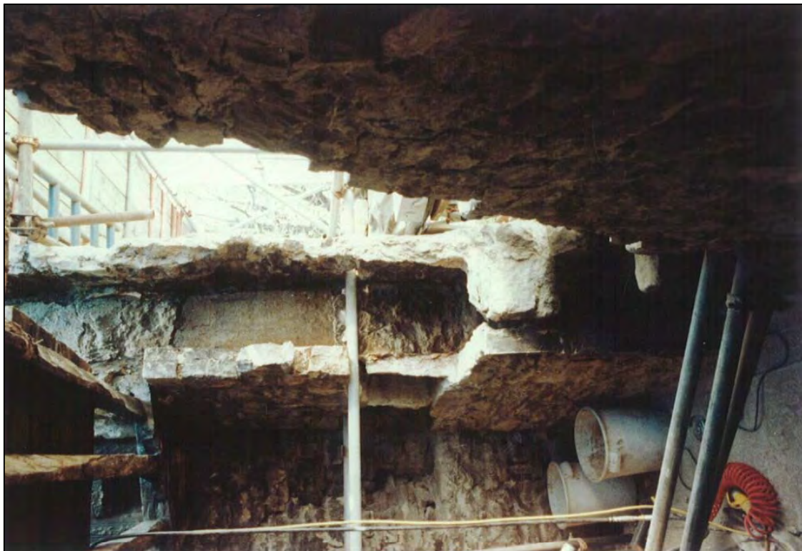
The south side wall was found to be unsafe and had to be rebuilt
